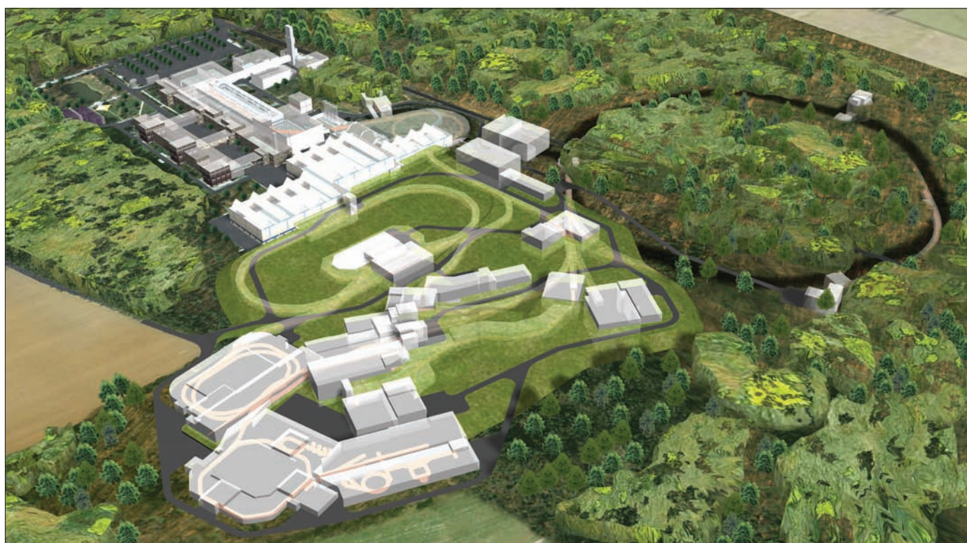
Fig.1. Artist's view of the Facility for Antiproton and Ion Research. The synchrotrons on the right will be 10–13 m underground.
